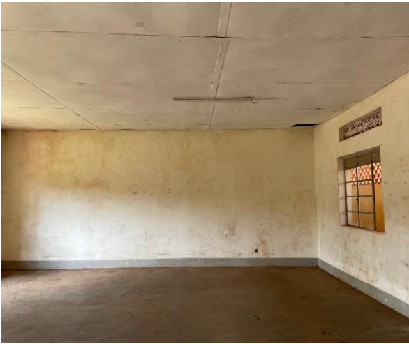
Girl's dormitory empty and ready to paint
